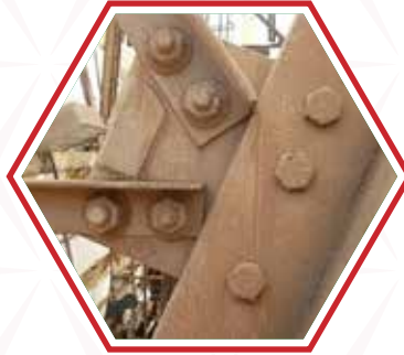
Derrick Bolts Tightening & Replacement
