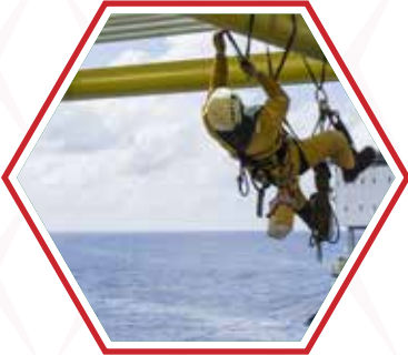
Rope access & Safe working at heights
